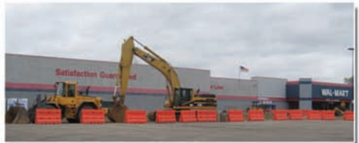
Super Walmart Building Project
