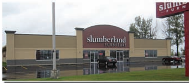
NEW Renovation of Slumberland
